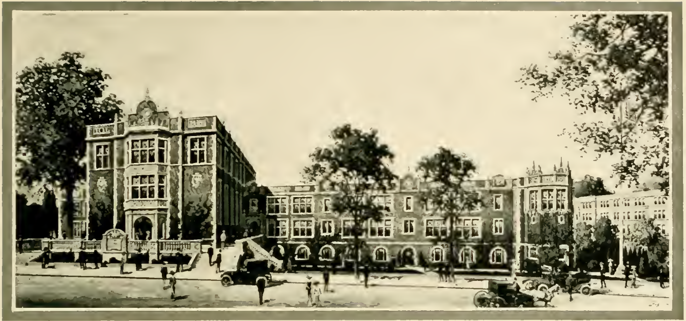
NEWARK NORMAL SCHOOL, IN COURSE OF CONSTRUCTION.
